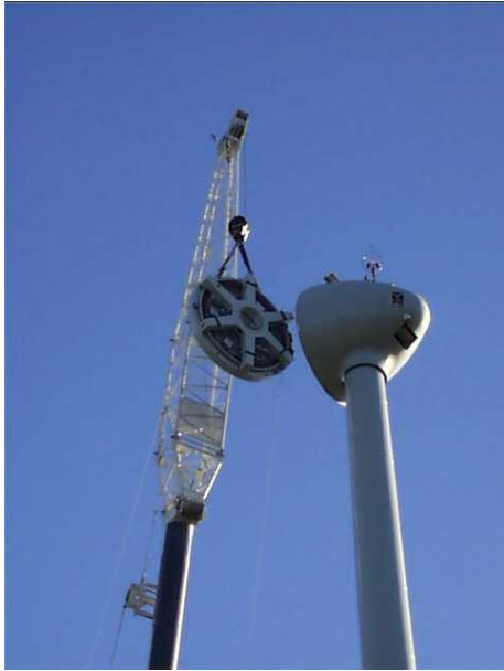
Joonis 1. Tuuliku generaatori montaaž Virtsus Figure 1. Installation of the generator to the wind-turbine in Virtsu
