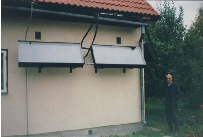
Foto 1. P. Voldi ehitatud soojaveekollektor. Photo 1. Home made solar-thermal collector.
