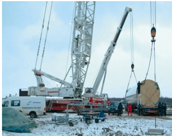
Joonis 2. Tuuliku monteerimine Pakri poolsaarel Figure 2. Erection of a wind turbine on the Pakri peninsula
