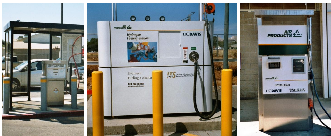
Figure 2.6. Filling units of methane, hydrogen and hythane at campus of University of California, Davis.
