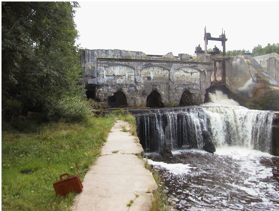
Figure 2. Linnamäe, a year before the rehabilitation
