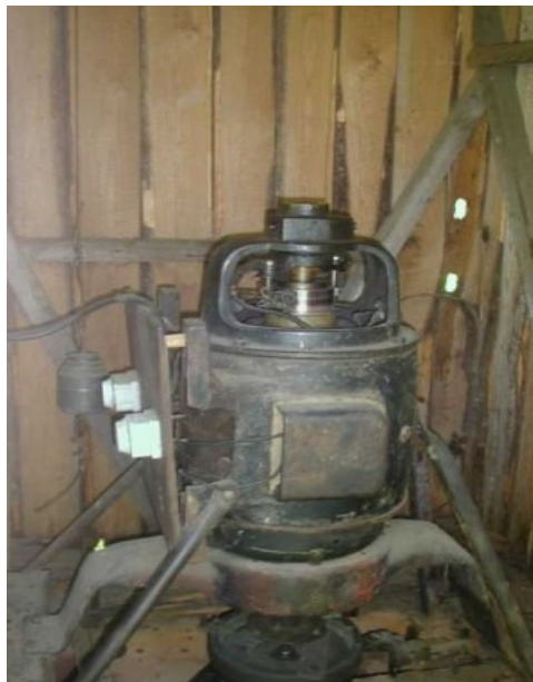
Joonis 2. Alalisvoolugeneraator Tindioru talus Figure 2. Direct current generator in Tindioru farm
